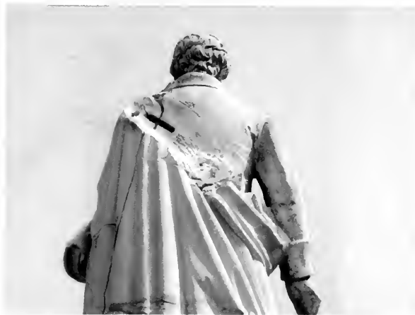
Figure 30: The figure of Father Mathew has missing parts, cracks and incompatible repairs (Photograph by author, March 2002)
